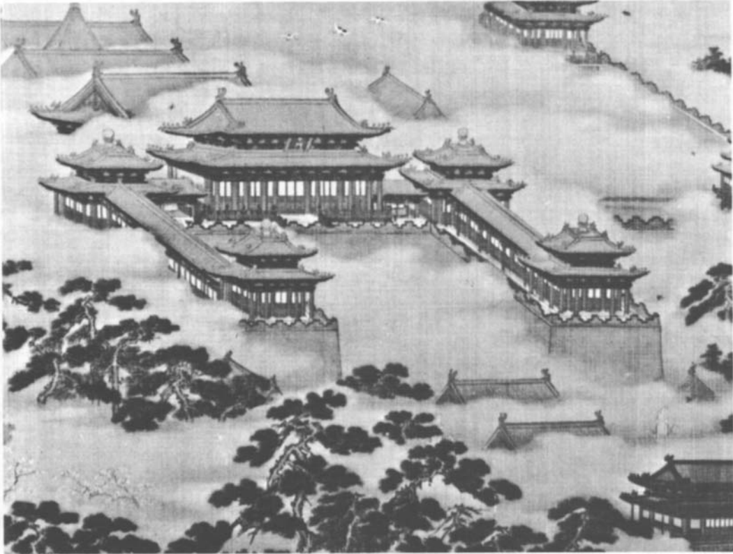
The Meridian Gate (Wu Men), main entrance to the Forbidden City.
